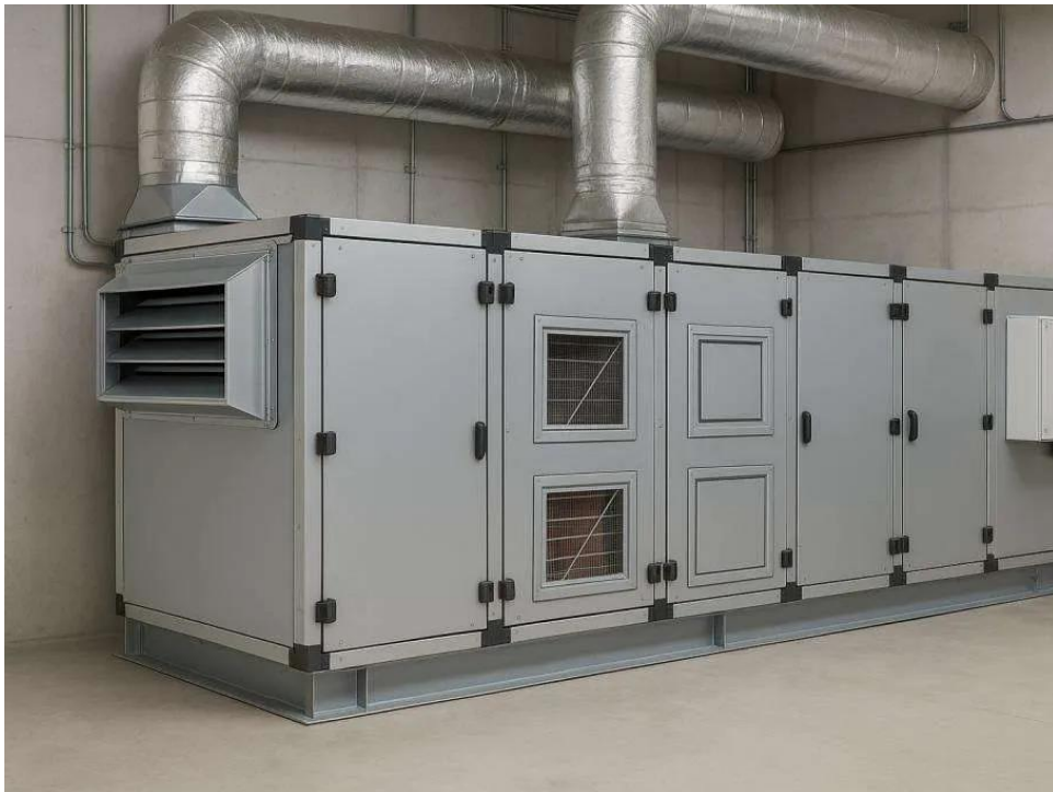
AIR HANDLING UNIT
